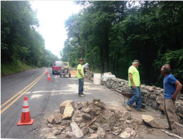
In addition to the improved road surface and new walking and biking paths, much of the historic stone wall was also repaired. A permanent plaque was installed along the roadway which will forever acknowledge the fine work and craftsmanship of the Eshbach Brothers who were actually part of the original construction of the stone wall back in the 1930's.
